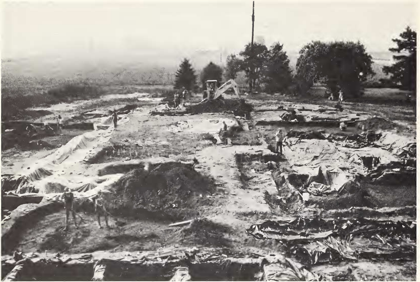
Fig. 1.2 General view of excavations, 21 July 1977. View looking south.
